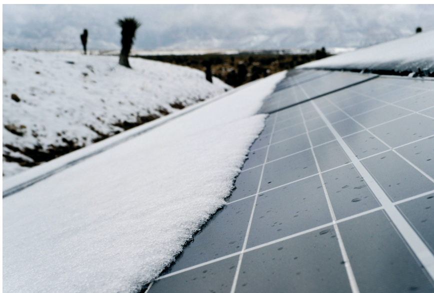
Figure 2. Snow acts as a serious source of shading.
